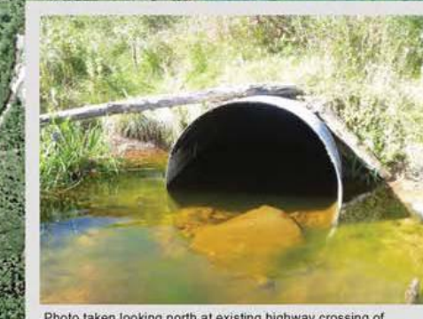
Photo taken looking north at existing highway crossing of Tributary F.
