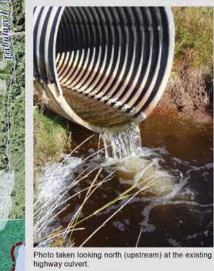
Photo taken looking north (upstream) at the existing highway culvert.
