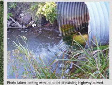
Photo taken looking west at outlet of existing highway culvert.
