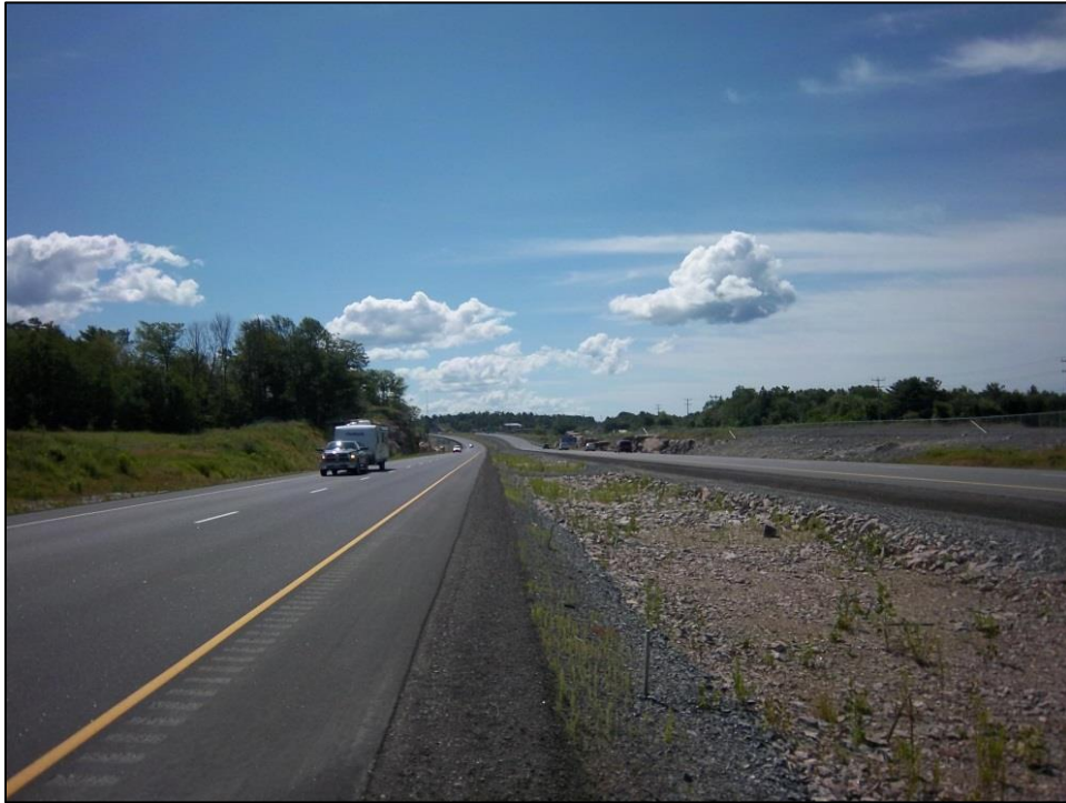
Example of a Four-Laned Highway 11/17
