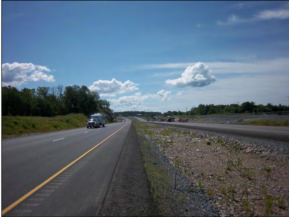
Example of a Four-Laned Highway 11/17
